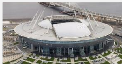
Gazprom Arena Saint Petersburg, Russia
